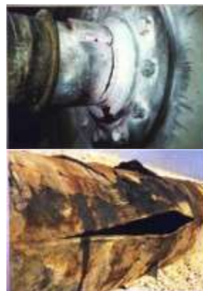
Failure cases in power stations
